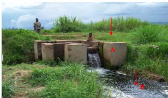
Photo4: Stream regulators Foreground B: canal A: Dam
