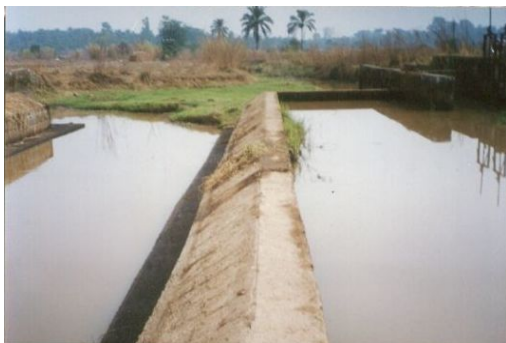
Photo3: Dykes to regulate water flow. Source: Mphoweh 2005
